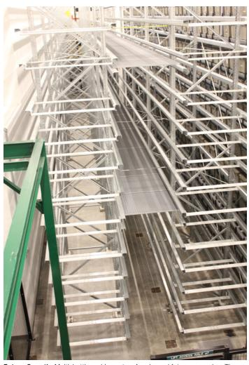
**Future Growth:** Multishuttle racking set up for planned future expansion. The modular design and scalability of the Dematic system allows capacity to be easily added.
